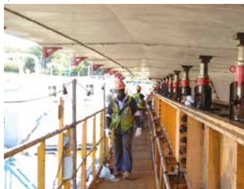
(42) HLN5508 lock nut cylinders lifting the Jordan Bridge in Chesapeake, VA.
